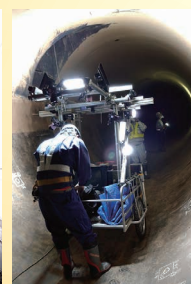
Water supply canal
